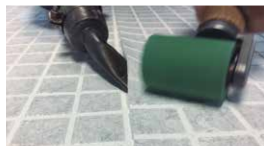
Overlap welded seams
