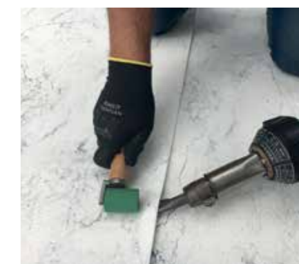
1 st Welding on the inside of the overlap
